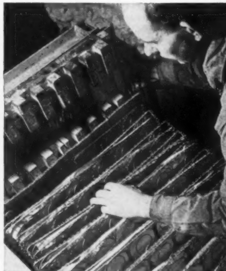
Baling for shipping, Piedmont upholstery springs are compressed to save space. Bill Gaston says, "We've never had a complaint from a customer because of the quality of the wire."
